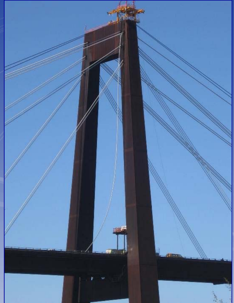
Extract de-tensioned existing stay
